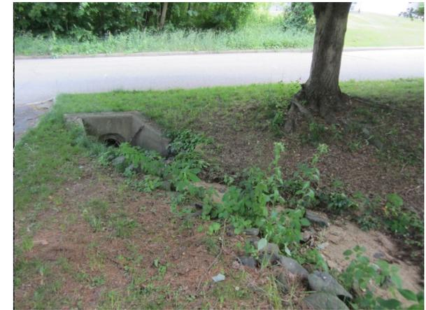
A small rain garden can be installed adjacent to the building to capture stormwater. Additionally, there is an existing drainage ditch on this site that is eroding. This could potentially be retrofitted into a bioswale, but more investigation is needed. A bioswale would prevent erosion, reduce pollutants, and enhance infiltration to the existing pathway. A preliminary soil assessment suggests that the soils have suitable drainage characteristics for green infrastructure.
